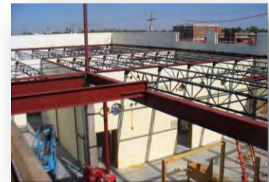
Interior ICF Studio walls under construction
