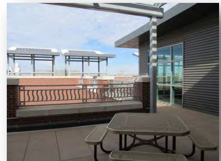
Second-floor Outdoor Patio
